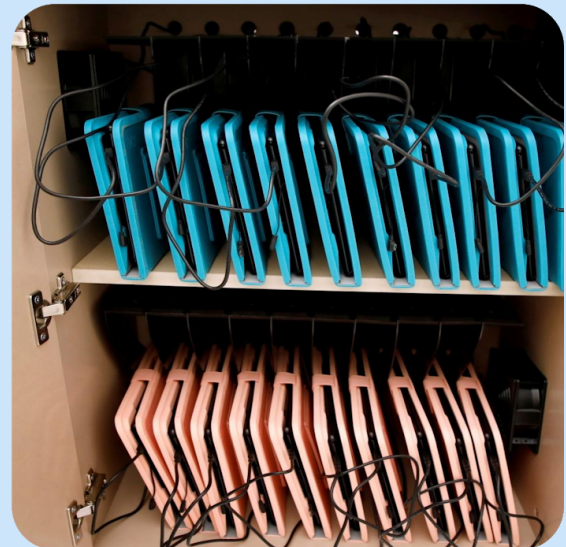
Cables Passed to Charging Compartment
